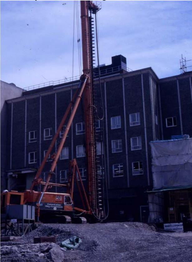
Figure 12. Continuous flight auger being used to install a 30 m bored pile for a new building foundation in central Shrewsbury, over a buried channel. © Copyright 2007 David Pannett
